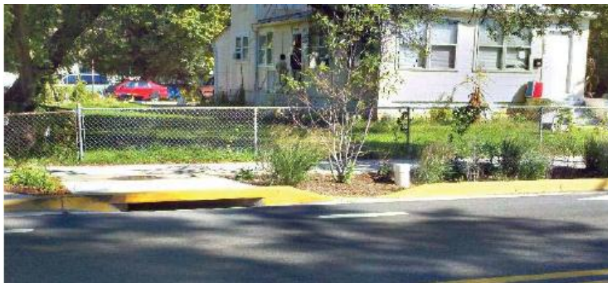
Decatur Street in Edmonston, MD utilizing both green and gray infrastructure. Photo courtesy of the Town of Edmonston, MD
