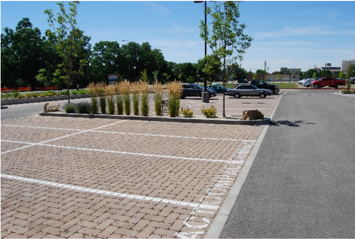
Photo credit: Tetra Tech, Inc. Figure 12. Private interests in Boise have adapted permeable pavement into parking systems
