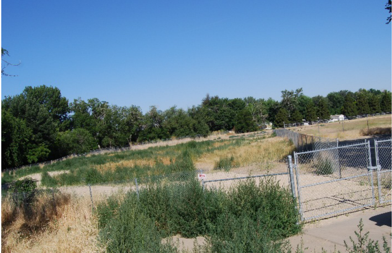
Figure 10. Infiltration basins often become overgrown with weeds and other vegetation
