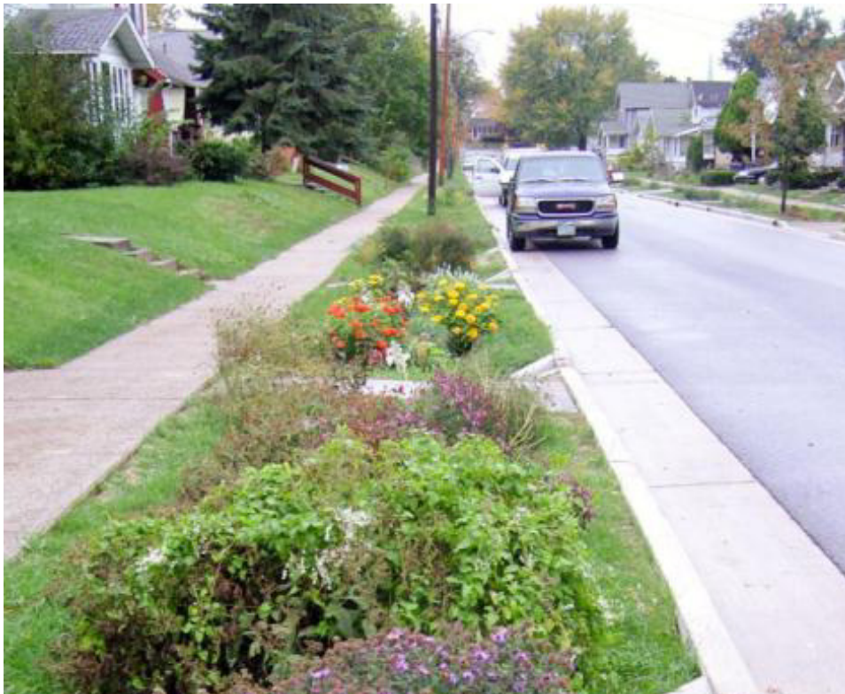
Figure 16. Bioretention integrated within a right-of-way vegetated fringe
