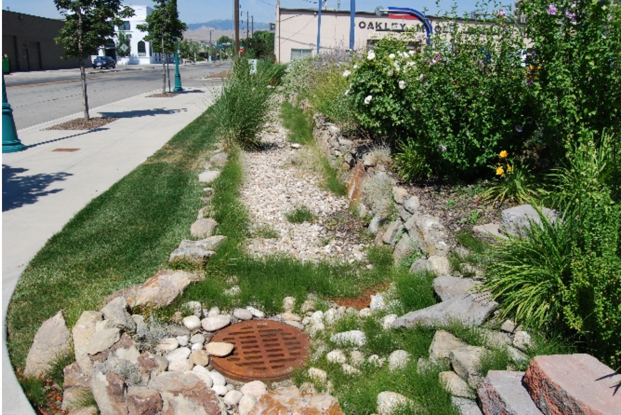
Figure 14. A bioswale along N 14 th Street provides stormwater management for a commercial carwash
