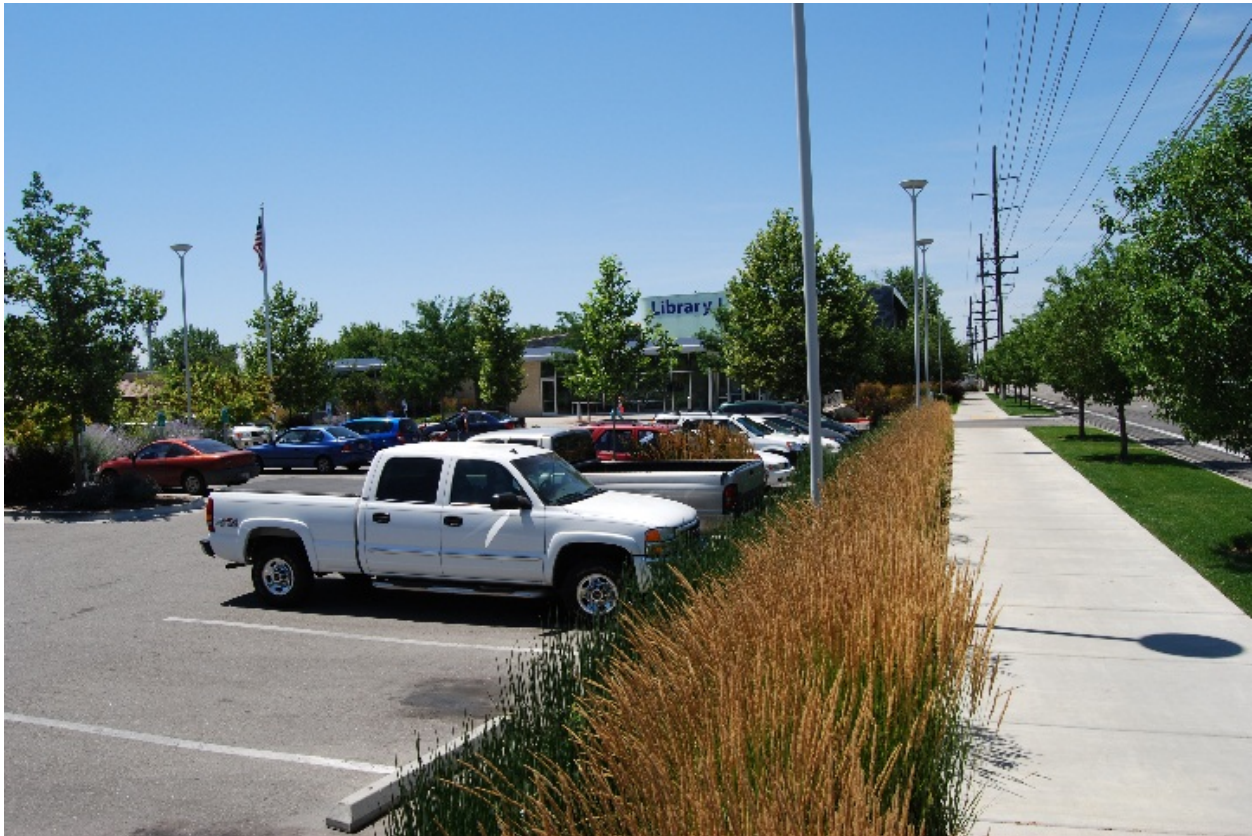
Figure 13. Bioretention located in a parking median at the Ustick Library
