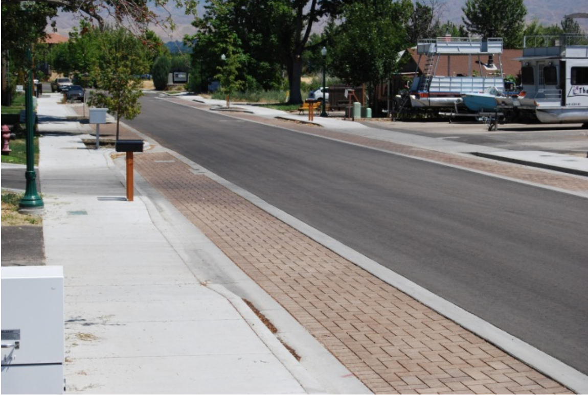
Photo credit: Tetra Tech, Inc. Figure 11. Permeable paver side street parking installed on 36 th Street, Garden City, ID
