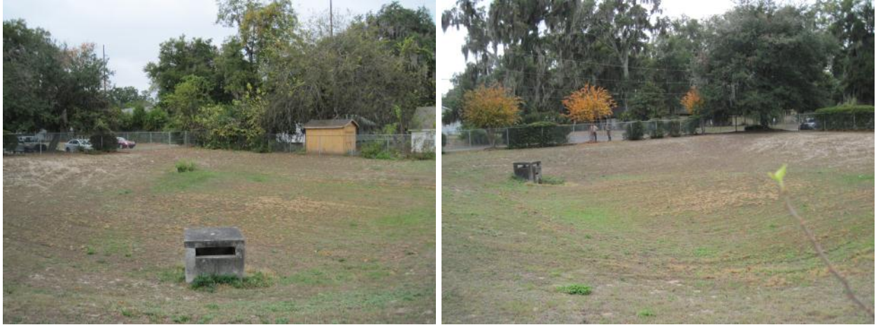
Figure 8. Dry pond at Hamar and Washington Streets.
