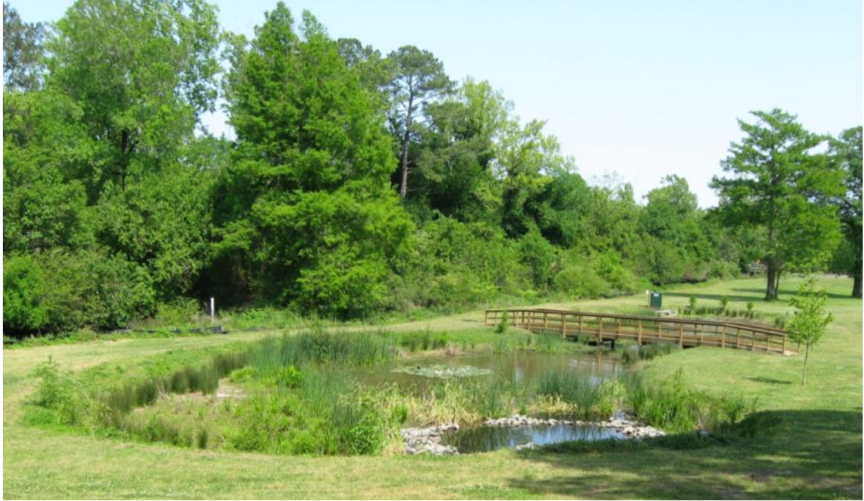
Figure 10. Example stormwater wetland.
