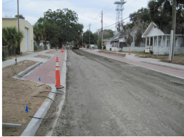
Figure 2. Green street construction on Duke Street.
