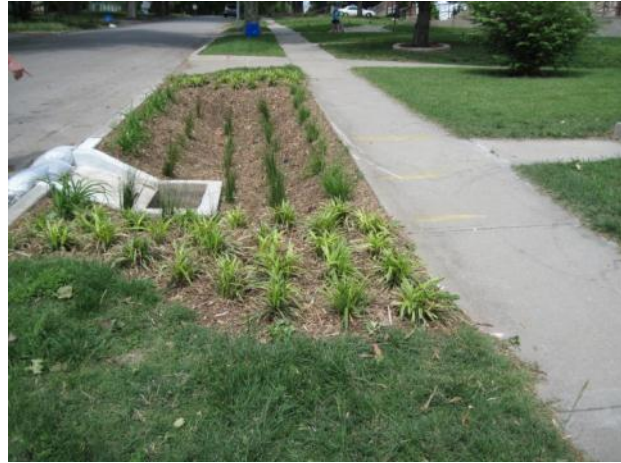
Figure 4-2. Bioretention incorporated into a right-of-way.
