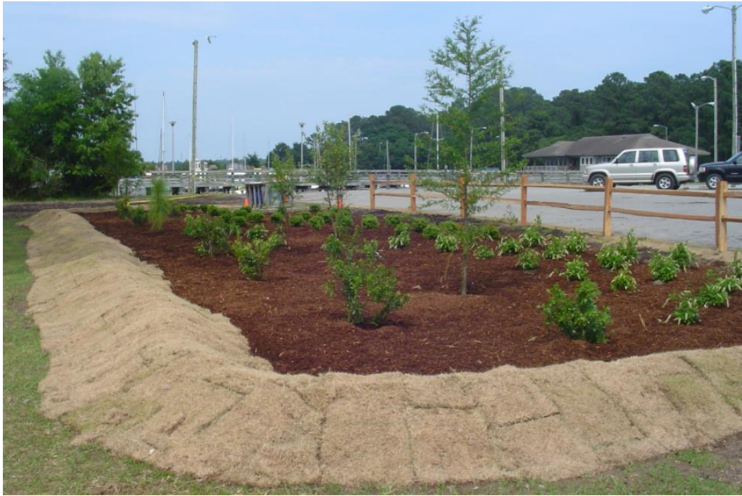
Figure 9. Example bioretention area.
