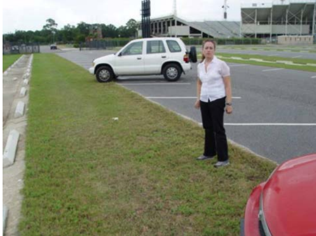
Figure 4-4. Grass paver parking stalls.
