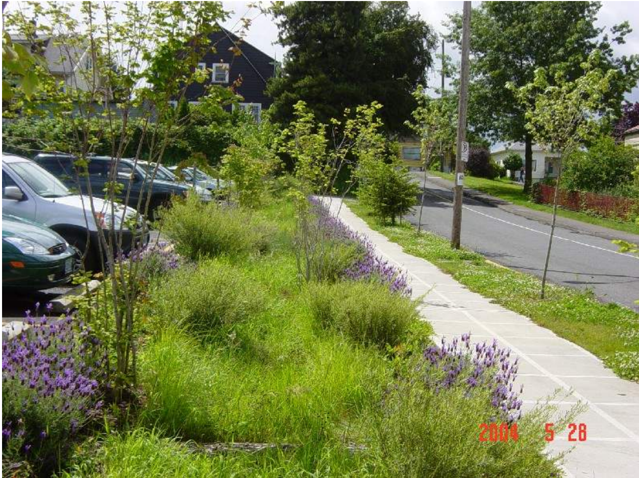
Figure 7. Example of a bioswale in the right-of-way.
