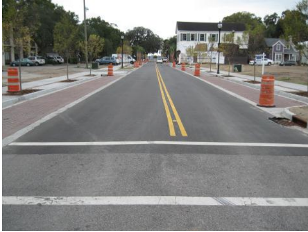
Figure 1. Permeable pavement on Bladen Street.
