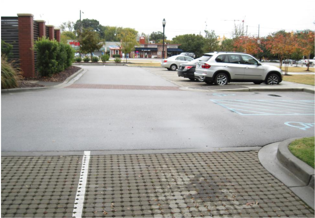
Figure 11. Permeable pavement parking stalls.
