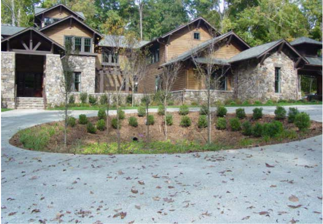
Figure 12. Residential bioretention with permeable pavement.
