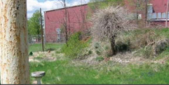
The Maytag Corporation's Dixie-Narco site is shown here prior to repurposing as the Ranson Civic Center.
