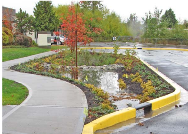
Trent Street Rain Gardens, Victoria, BC, Canada. Courtesy of Murdoch de Greeff Inc.
