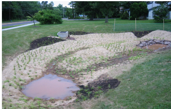
Constructed Wetland Designed by F.X. Browne, Inc.
