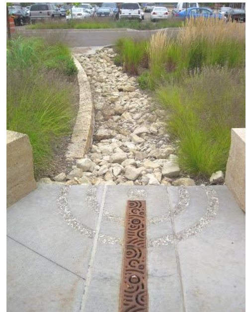
Drain collects runoff from impervious surface and directs it to rain gardens in Saint Paul, MN.
