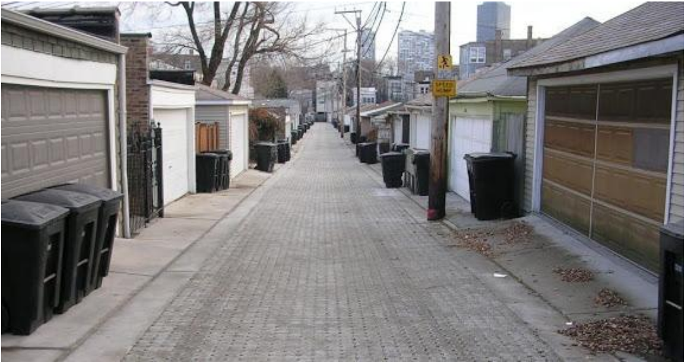
Photo: Permeable paver retrofits help to infiltrate urban runoff in a Chicago alley. © Abby Hall, U.S. EPA.
