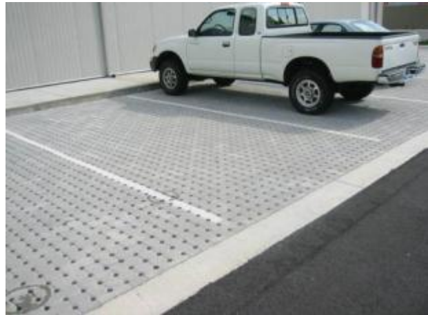
Figure 4-4. Permeable Interlocking Concrete Paver Parking Stalls
