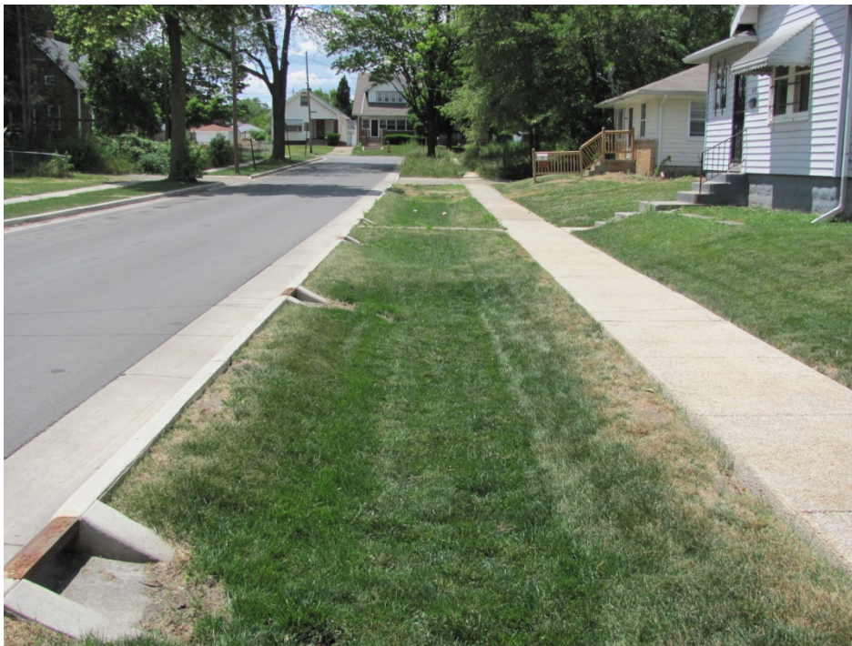
Figure 6-1. Bioretention Planted with Turf Grass
