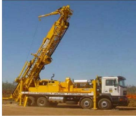
Exhibit 16: Slant hole drilling [Mitchell Drilling, 2005]
