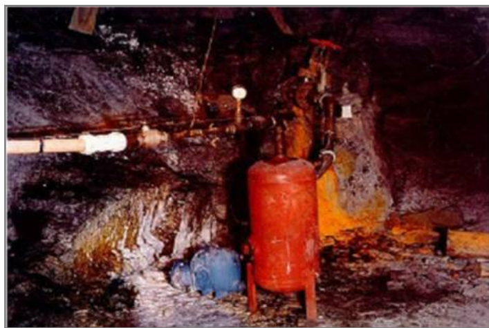
Exhibit 30: Separation system at the base of a vertical collection well
