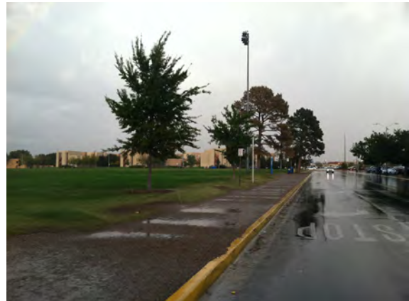
Ponding and washout on jogging path 9.30.2017
