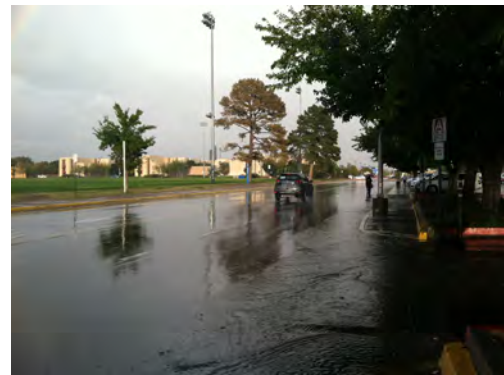
Flooding on Redondo Drive 9.30.2017
