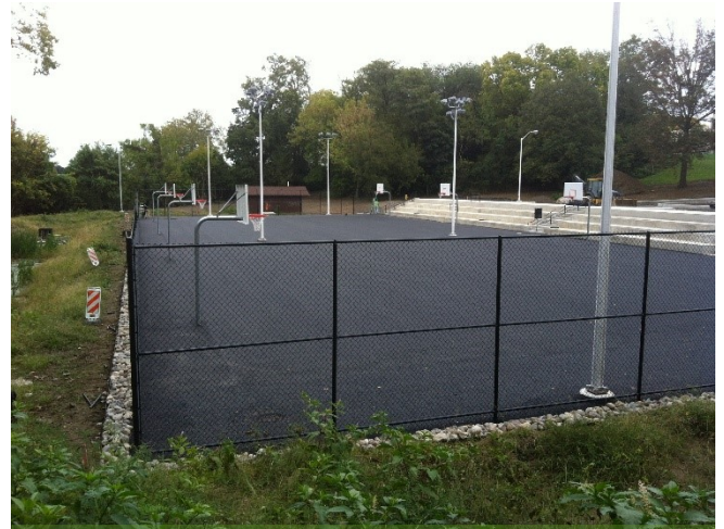
Lancaster City's Brandon Park is home to a basketball court constructed over permeable macadam, allowing stormwater to infiltrate into the soil underneath the playing surface. (Photo courtesy of the Lancaster City Department of Public Works)
