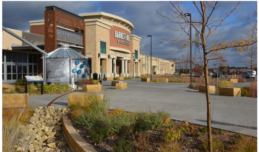
A bioretention installation helps manage stormwater runoff from adjacent streets and sidewalks. (Photo courtesy of the Ramsey-Washington Metro Watershed District)
