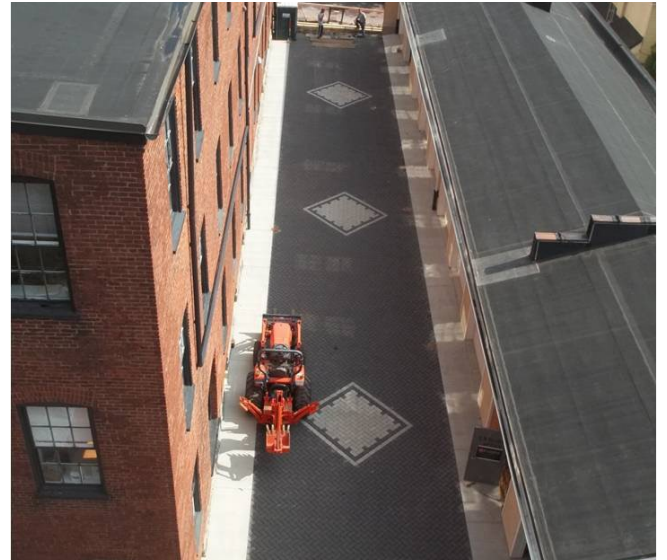
Permeable pavement lines an alley in downtown Lancaster City. (Photo courtesy of the Lancaster City Department of Public Works)
