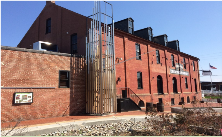
A 750-gallon cistern and bioretention basin outside of the Lancaster Brewing Company. (Photo courtesy of the Lancaster City Department of Public Works)
