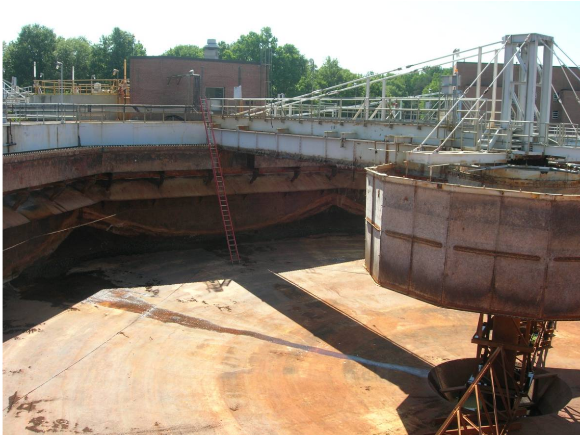
Empty tertiary clarifier at Noman Cole PCP
