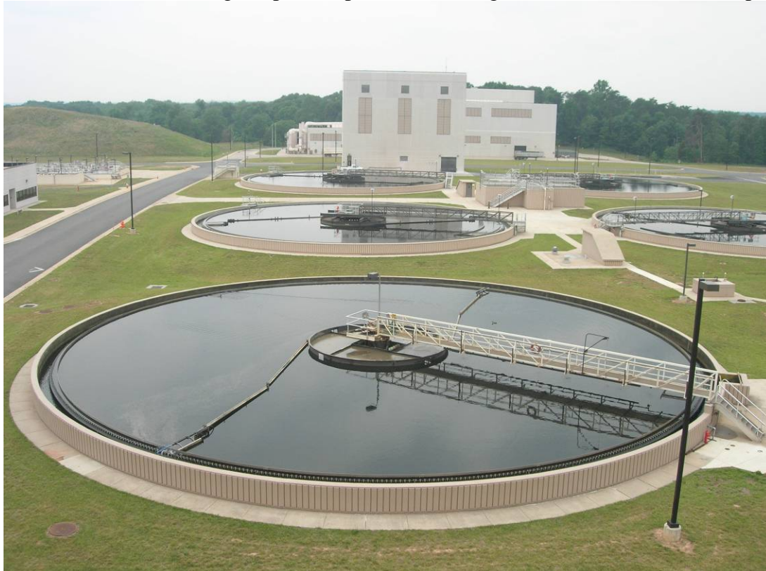
Secondary Clarifiers with lime handling buildings in background at UOSA WRF
