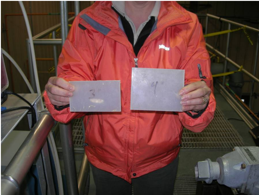
Plastic weirs used for adjusting overflow rate from DynaSand Filters
