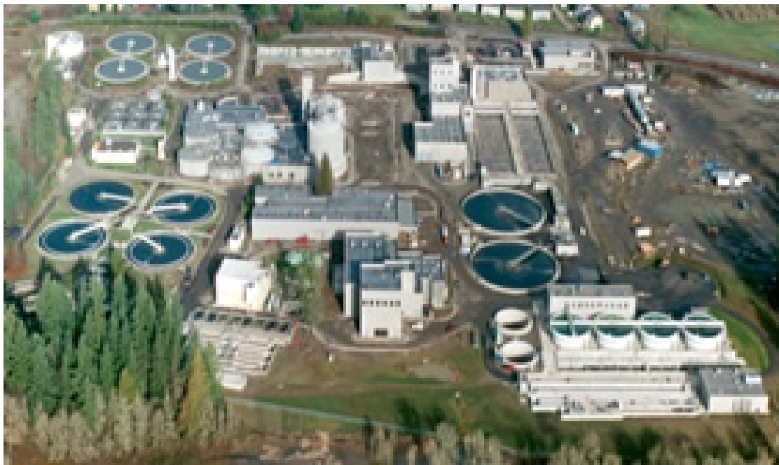
Clean Water Services Rock Creek AWWTP (from CWS informational publication)
