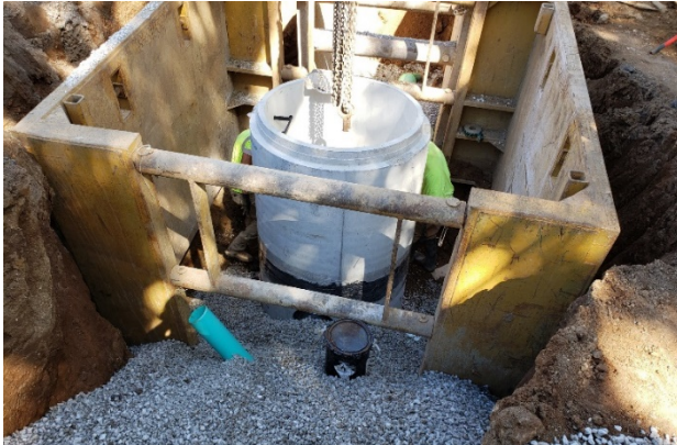
Photo #1: View of the installation of new sewer manhole #250051
