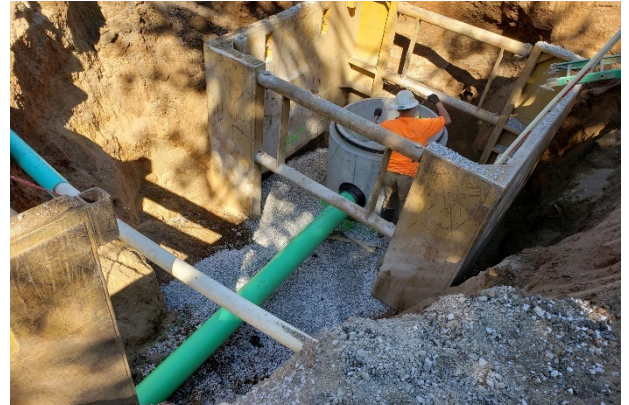
Photo #2: View looking west at newly installed manhole #250052
