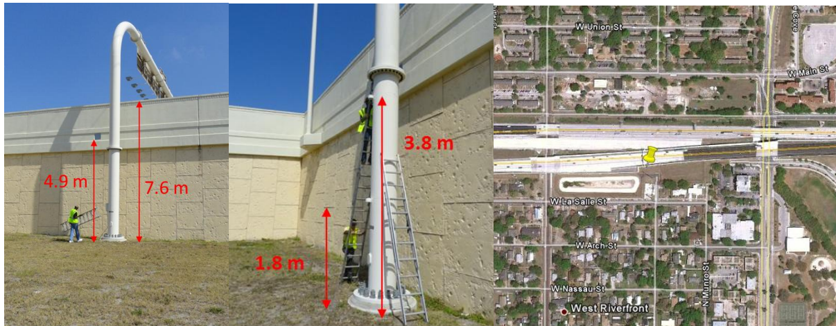
Figure E-5. Tampa EPC03 site photos (left and middle) and Google Earth image (right). Site is an elevated road (4.9 m agl) with a safety barrier (2.7 m). The top of the wall is 7.6 m above grade level. The PSD mounts are 7 m from the travel lane in the horizontal and 3.8 m and 5.8 m below the wall.
