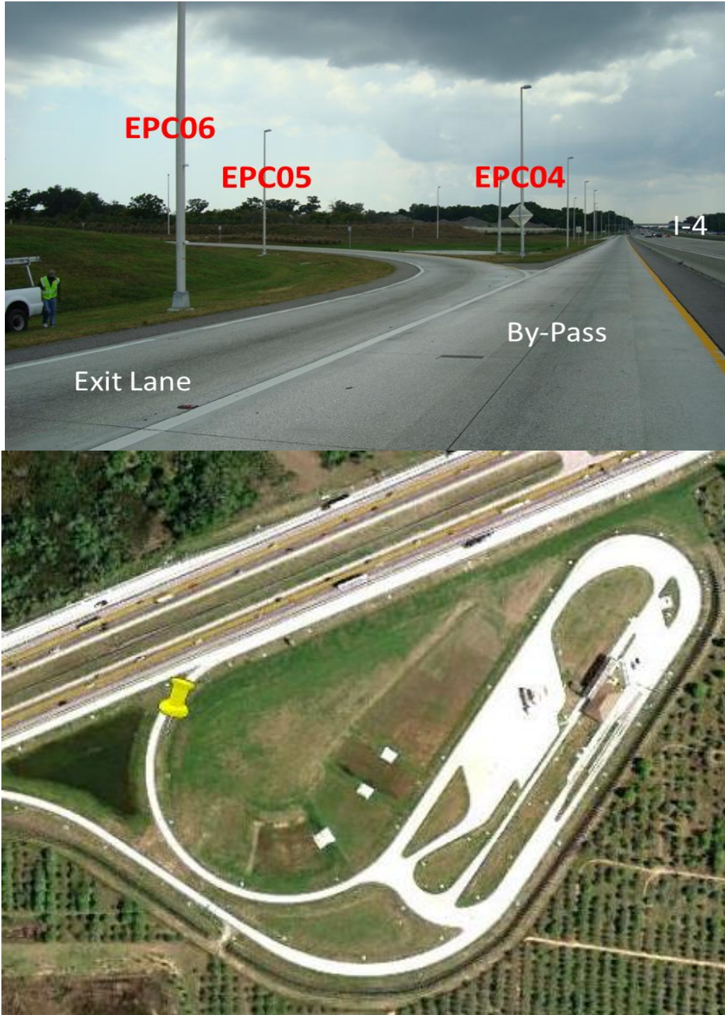
Figure 3-3. Tampa EPC04, EPC05, and EPC06 site photo (top) and Google Earth image (bottom). This was the transect location. In the top photo, the lanes from left to right are the weigh station exit, the bypass lane, and the I-4 travel lane.
