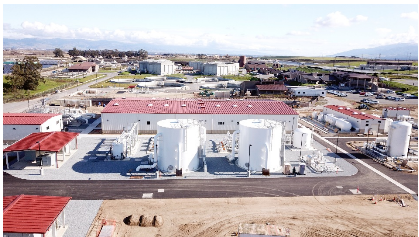
Pure Water Monterey (CA) potable reuse facility
