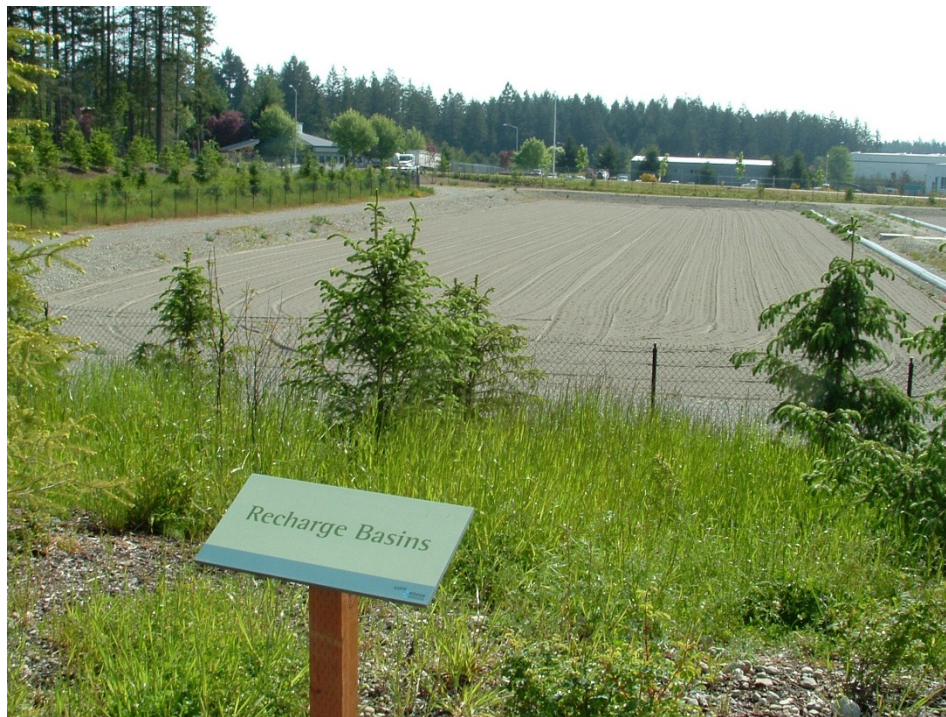
Hawks Prairie Ponds and Recharge Basins (LOTT Clean Water Alliance, WA)
