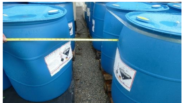
Insufficient aisle space between chemical drums.
