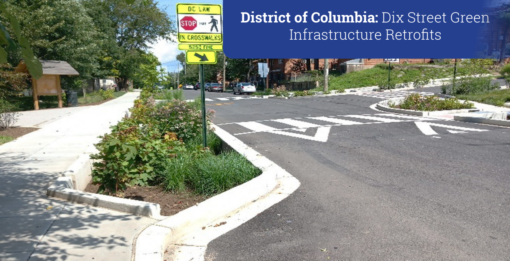
Bioretention Bulbouts at Intersection of 53rd and Dix Streets NE
