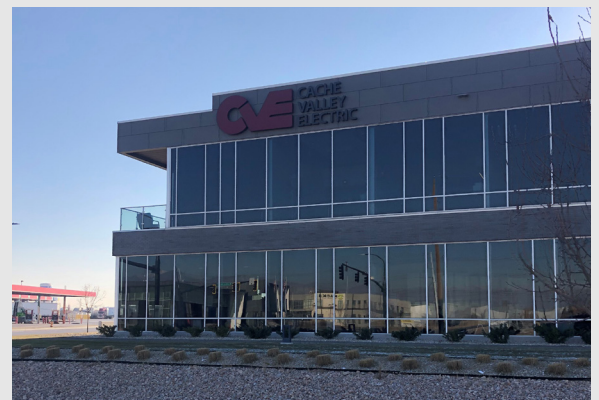
Cache Valley Electric is one of the site's largest businesses, with more than 130 employees.
