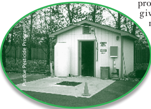
Maintain a well designed, secure pesticide storage facility with highly visible warning signs. Keep it well ventilated and located where water damage is not likely to occur.
