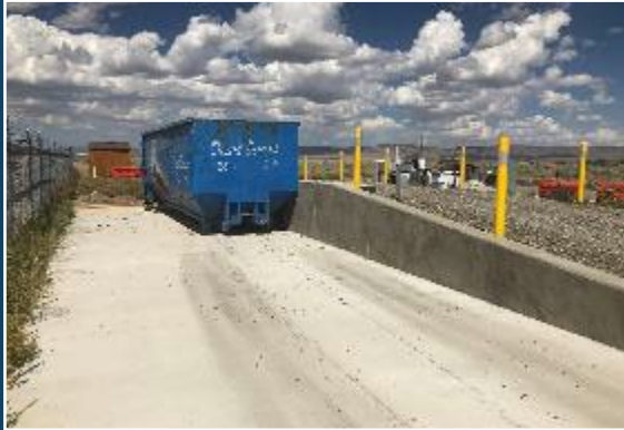
Cement Base under transfer bins, concrete and steel reinforced retaining walls.
