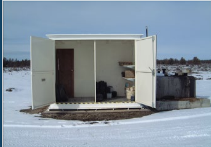
Small storage building and oil tank
