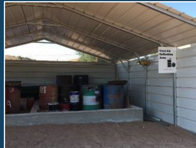
Carport with raised concrete pad for used oil collection
