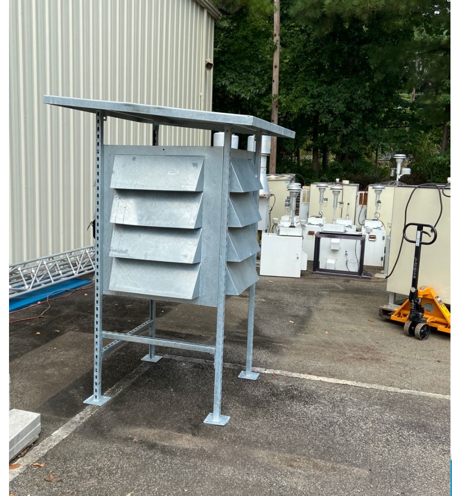
Collocation Shelter after construction in Raleigh, North Carolina
