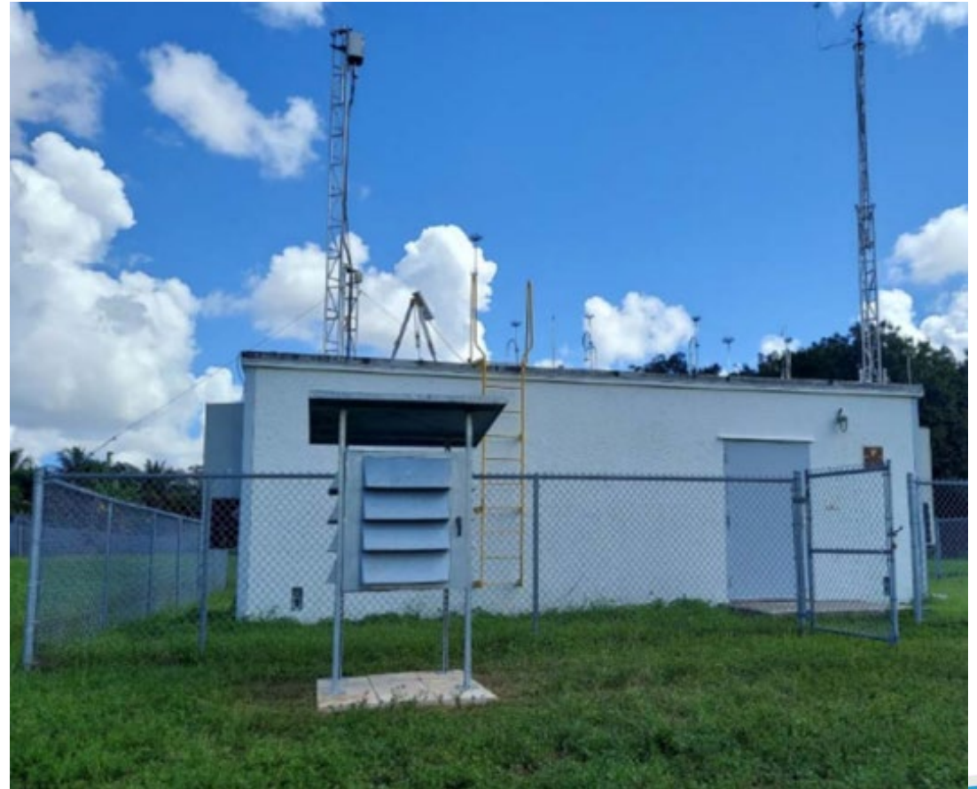
Collocation Shelter installed in Broward County, Florida
