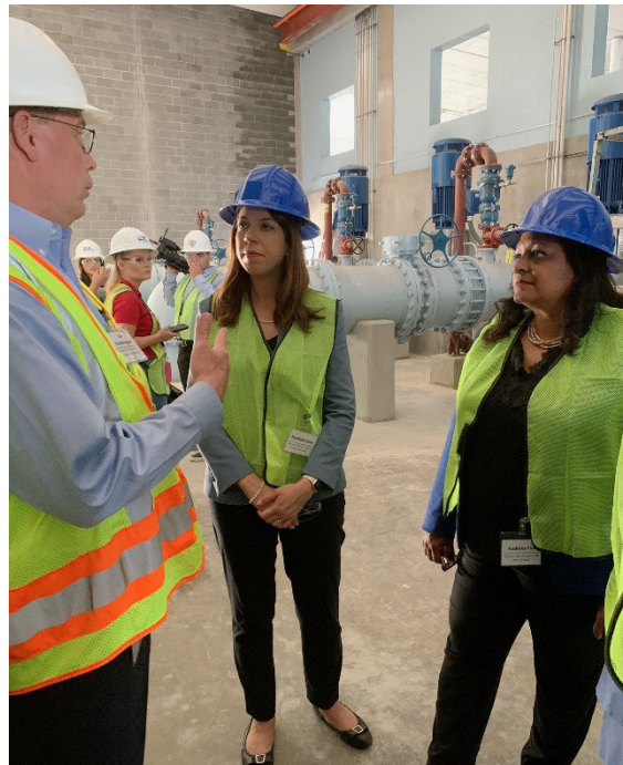
Radhika Fox, Co-Chair of EPA's PFAS Council and Assistant Administrator for the Office of Water, and Elizabeth Biser, Secretary of the North Carolina Department of Environmental Quality, tour a new Granular Activated Carbon system at the Sweeney Water Treatment Plant in Wilmington, NC, on June 15, 2022.
