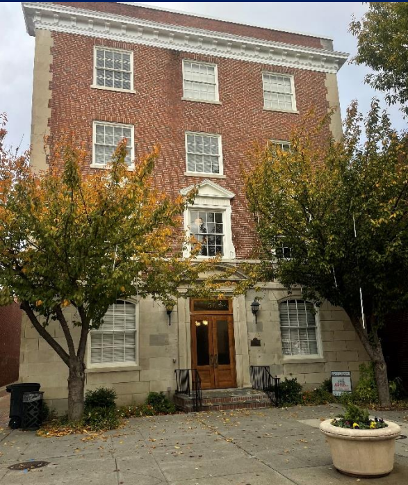
The Chief Tassel building opening in 2022 offering eight commercial office spaces and 18 apartments.
