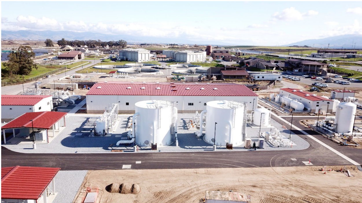
The Pure Water Monterey project in Central California uses municipal wastewater, stormwater, agricultural drainage, and agricultural wash water in its potable reuse facility to replenish the Seaside Groundwater Basin.
