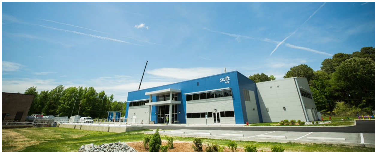
The Hampton Roads Sanitation District's Sustainable Water Initiative for Tomorrow will replenish the Potomac Aquifer to improve water quality in the Chesapeake Bay and mitigate land subsidence.
