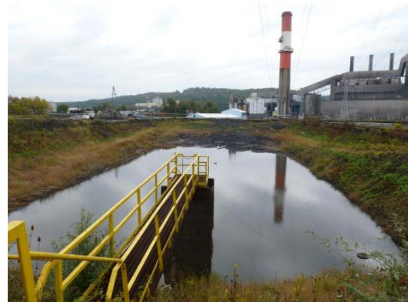
Surface impoundment at a coal-fired power plant.
