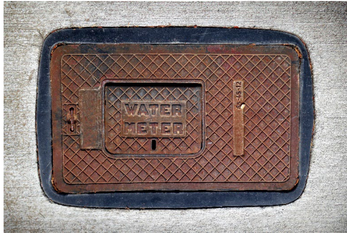
Water meter box cover
