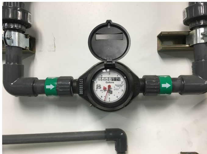
Submeter used to monitor reverse osmosis system
