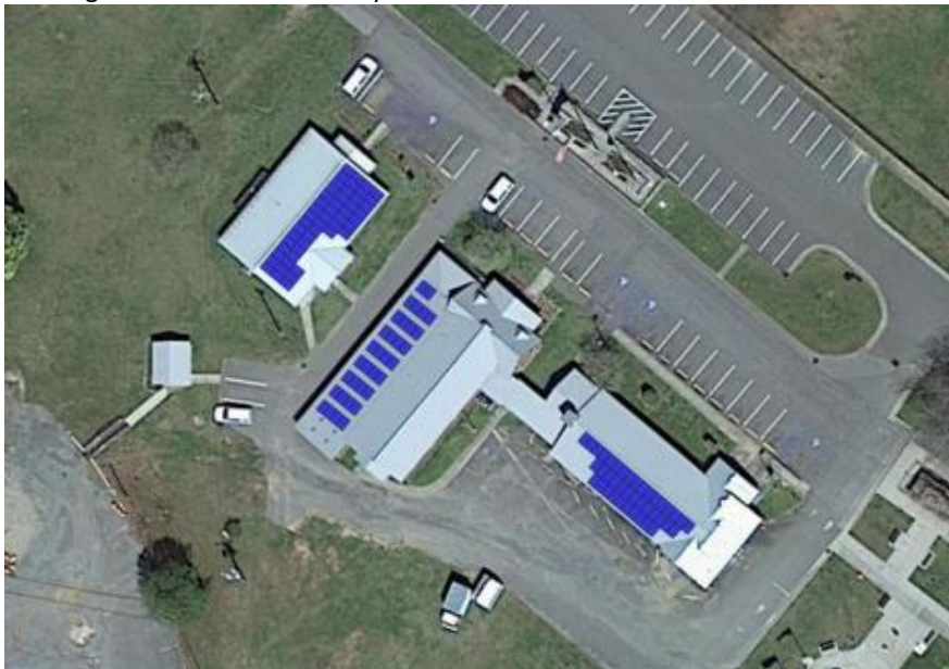
Figure 6. 124 solar panels, totaling 52.08 kW will be installed on the Tribal Council building on the Qualla Boundary.
