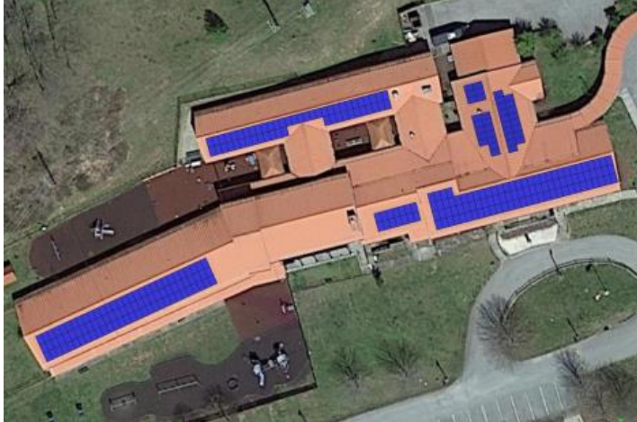
Figure 7. 288 solar panels will be installed on the new Kituwah Academy building.
